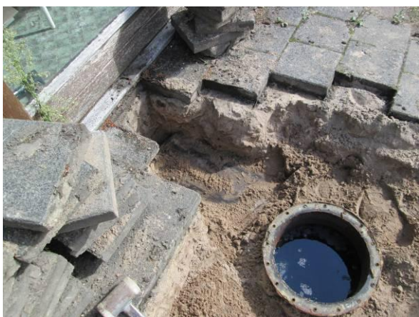
Foto 7: Mangat 30.000 liter petroleumtank
